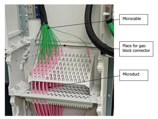
Fig.6. Microducts fixing and cutting to proper length.
