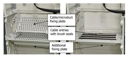
Fig.3, 4. Cable/microduct fixing plate and cable entries with brush seals
