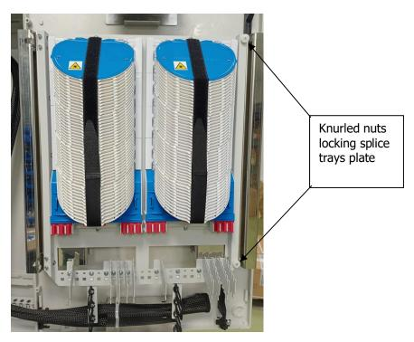
Fig. 2. Locks for opening the splice tray plate and disassembly of the inner box.
