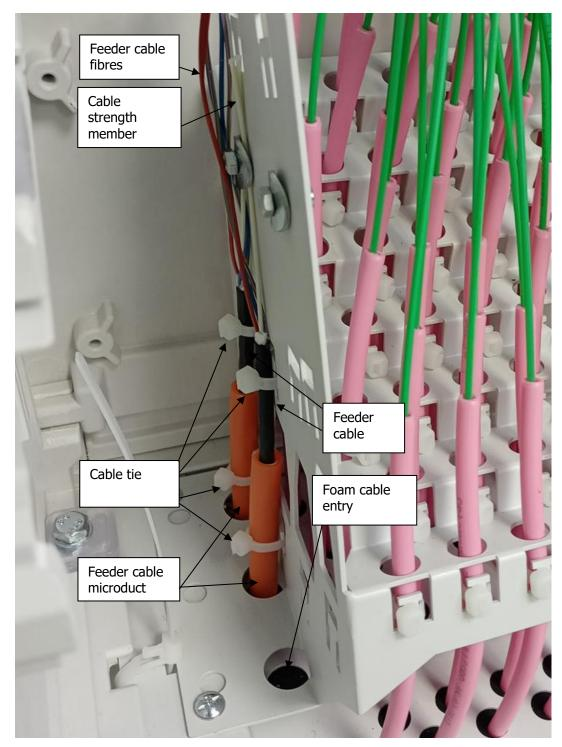
Fig.5. Microduct/cable entry into the cabinet.
