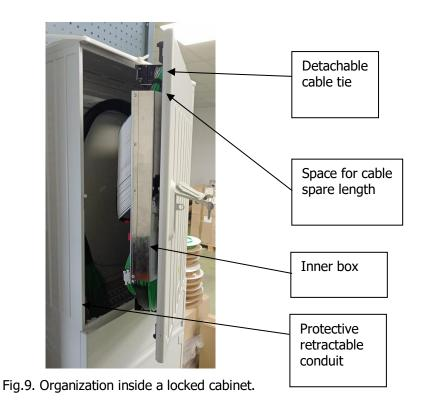
**Note 1:** Remove the front door to allow the inner box to be put on the ground to make splicing and maintenance works comfortable.
