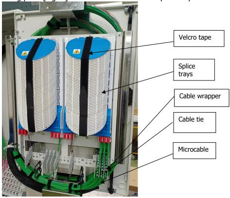
Fig.8. Routing cables to splice trays.
