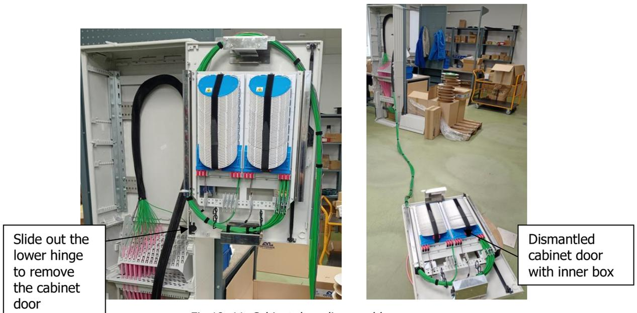
Fig.10, 11. Cabinet door disassembly
